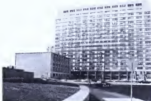
Labor and Industry Building; Indiana limestone exterior accented by vertical bands of Georgia marble; columns at main entrance, Minnesota "rainbow granite."
